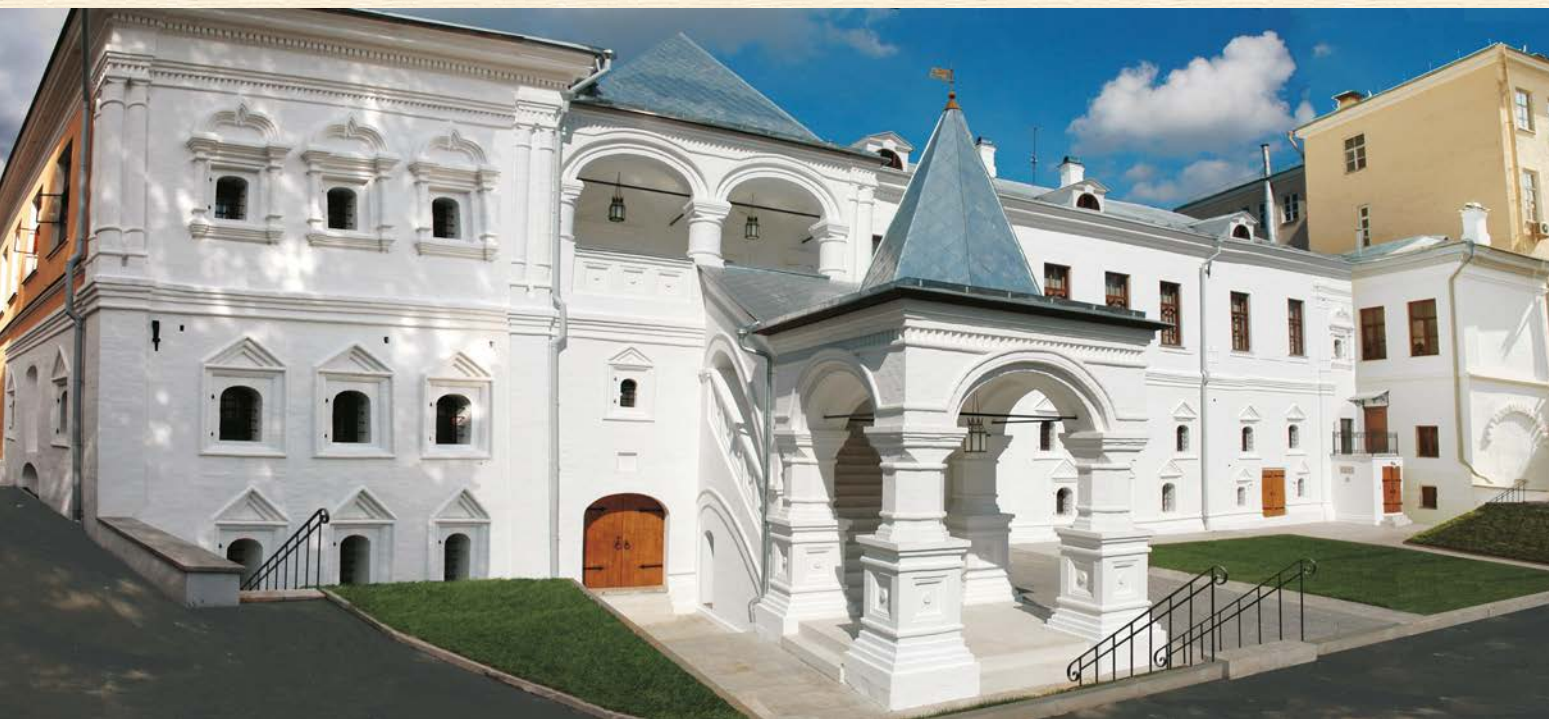
Yard facade panorama with the reconstructed 17 th century's Red porch upon the full completion of the restoration works, August 2006
