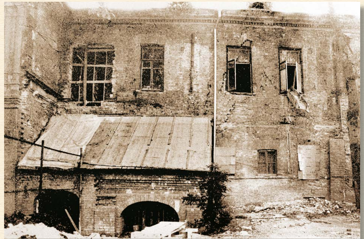
Central part of the yard facade, fragment, 1995
