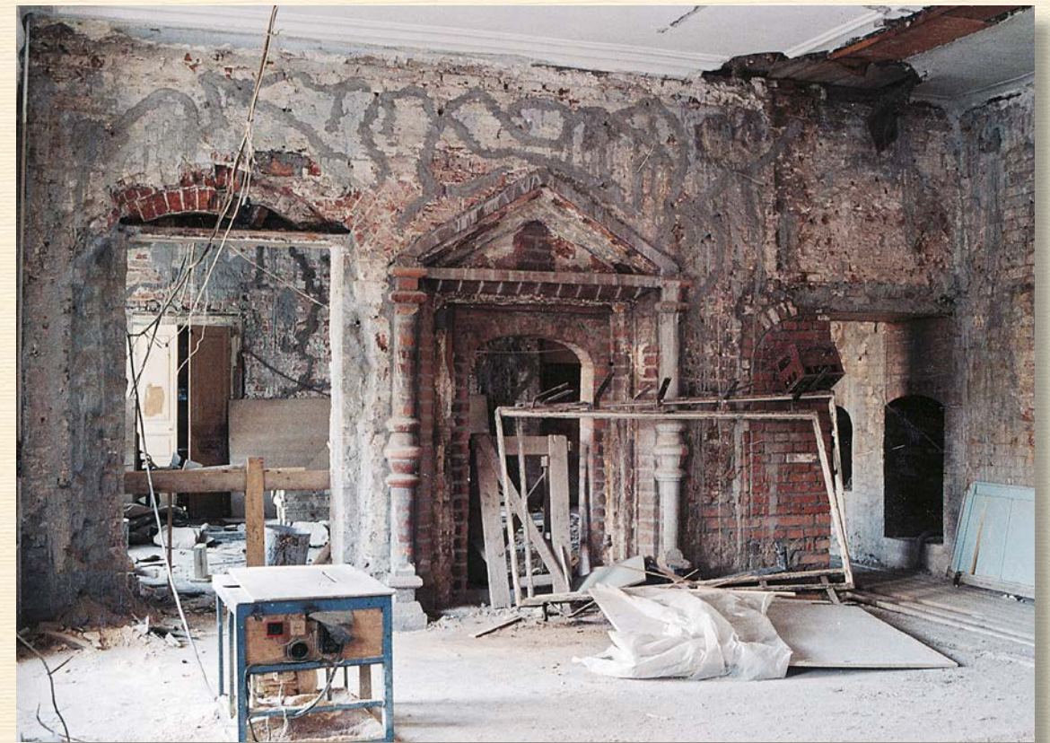
First floor east enfilade hall during restoration, 1995
