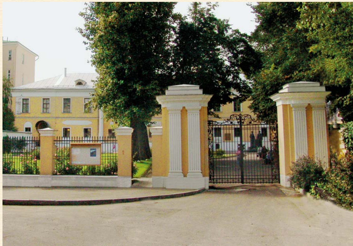
The original fencing was restored in 1997
