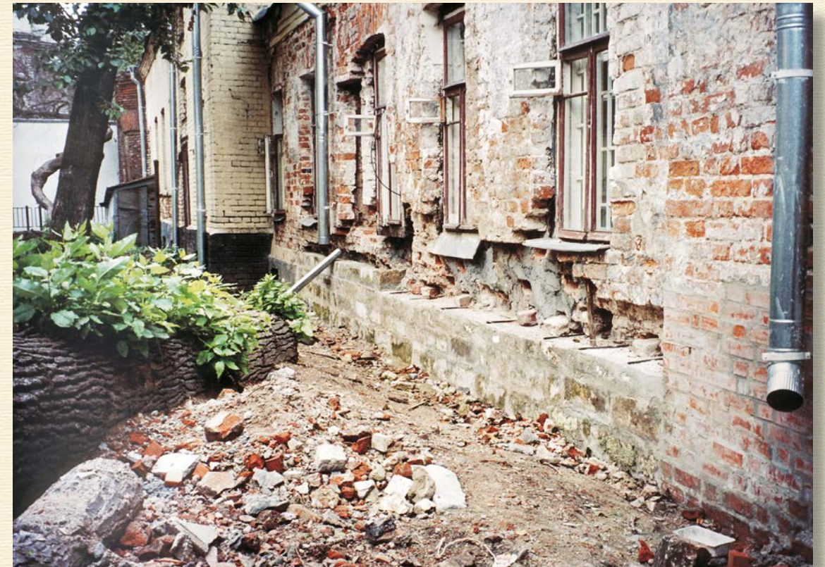
Yard facade during restoration, fragment, 2003
