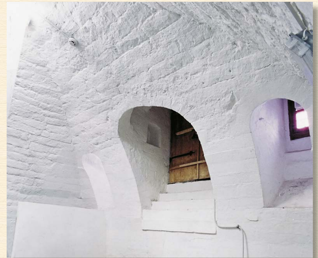
The central white-stone basement was restored in 2000–2001
