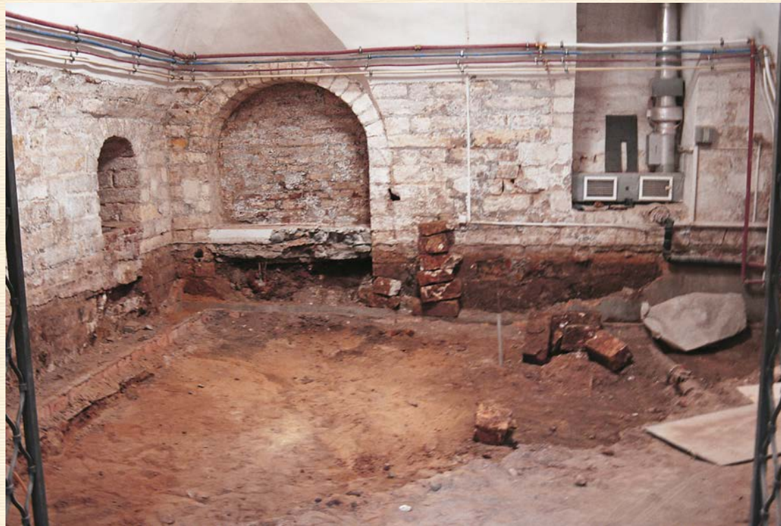
White-stone basement of the north risalit
